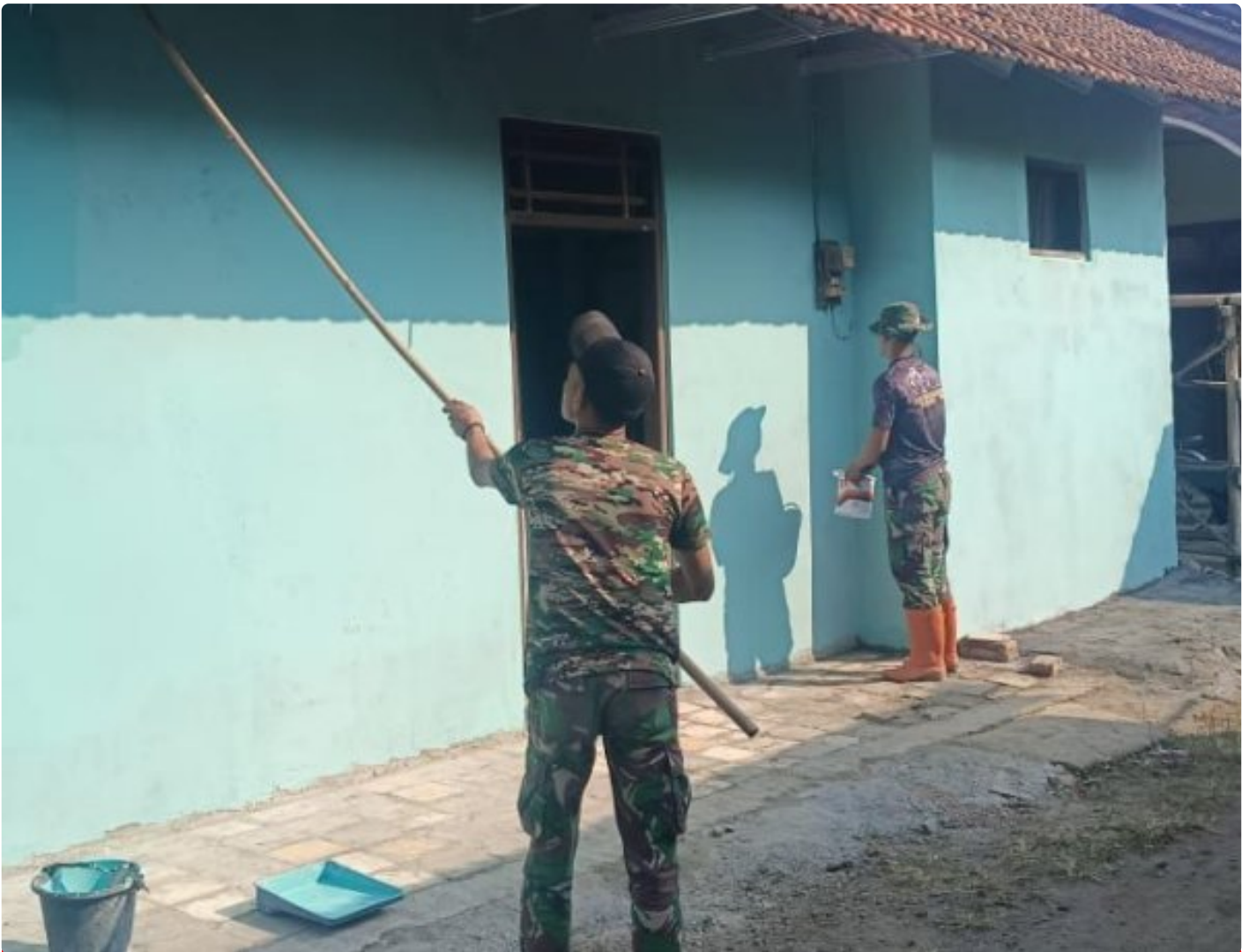
(Foto istimewa) Pengecatan RTLH TMMMD 116 Kodim 0722/Kudus
